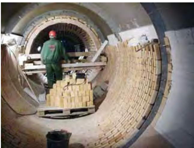
Installing Bjuf SX bricks in a TAD
